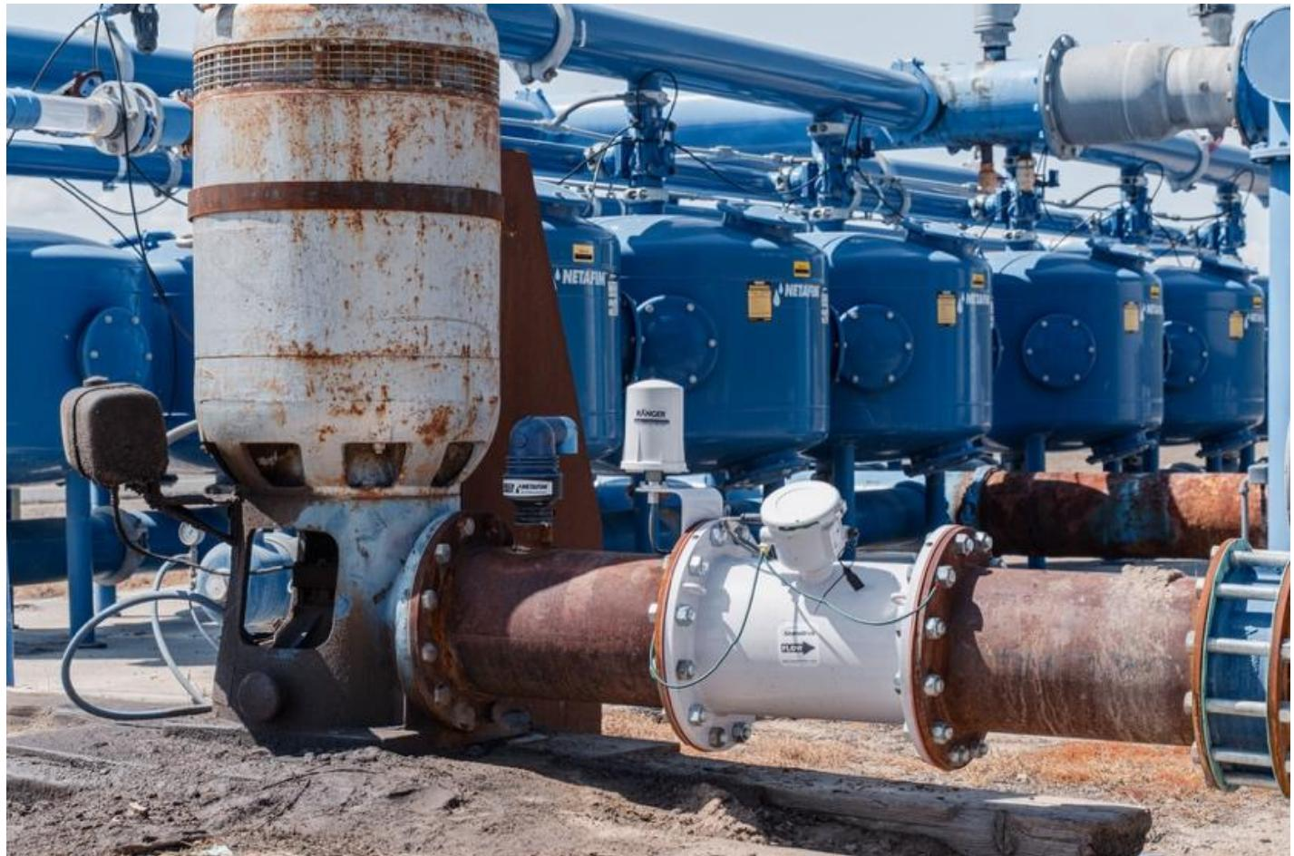
To wake the meter up, cover one of the arrows for 5 seconds and then uncover. If the meter does not wake up, follow that procedure again. To save battery life, the meter only looks for the switch input once every 5 seconds. The meter will probably wake up easier than this but may need the full 5 second inputs.
