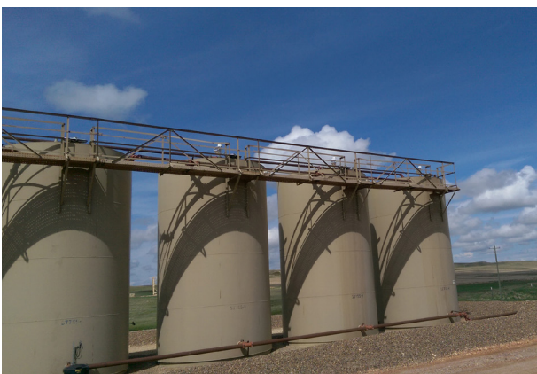
Figure 2. SignalFire Sentinel HART Wireless nodes with Class 1 Division 1 solar power provide wireless access to HART data from guided wave radar level sensors on these tanks.
