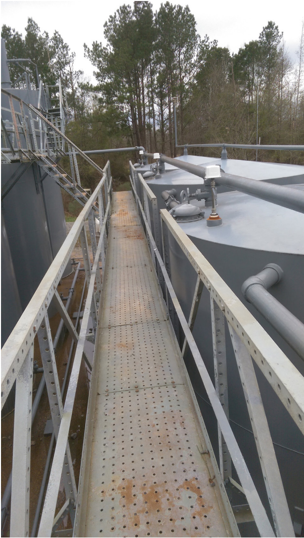
Figure 1. SignalFire Sentinel wireless nodes with Modbus interface to tank level float sticks. The node's internal batteries power both the sensor and radio, transmitting critical asset data that is used by the operator to monitor tank levels.
