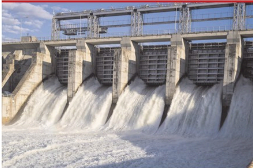
Traditional hard-wired monitoring systems can create reliability and cost challenges for operators, leading to increased interest in wireless options. Photo courtesy SignalFire Wireless Telemetry
