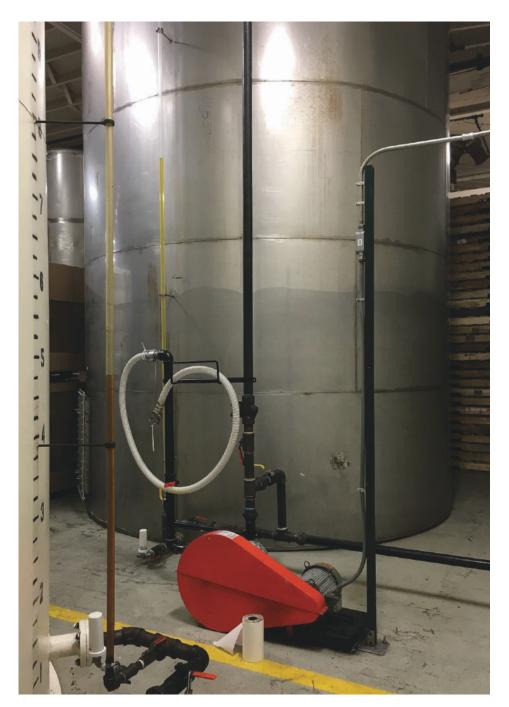
manufacturer of tortilla products utilizes large supplies of cooking oil as part of its production process of frying corn and flour tortilla chips. Two separate 20-foot tanks located inside the processing facility hold supplies of virgin and wasted cooking oil. Managing oil levels in these tanks is important to ensure when to order new supplies of cooking oil and dispose of the wasted stock.
